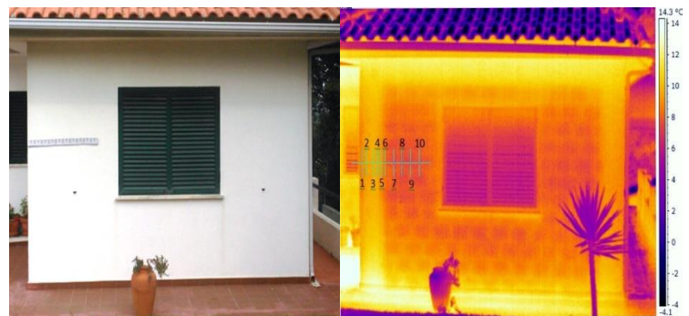
► Fig. 2: Façade of a single and its thermographic image [3].
