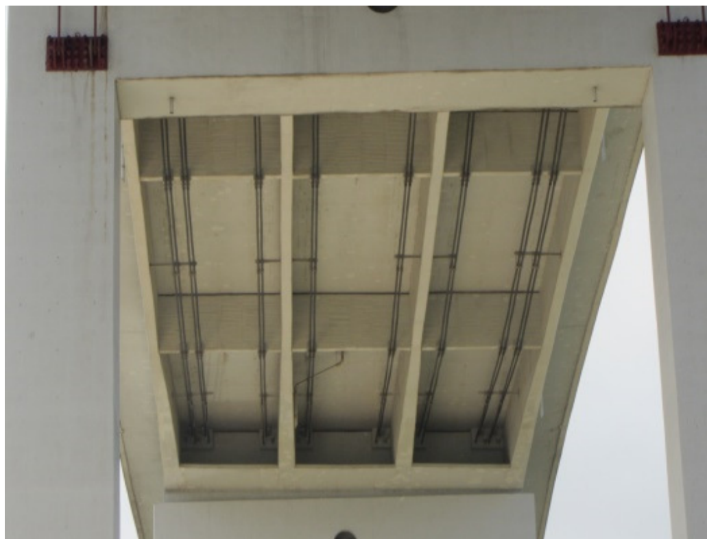
Fig.1: Externally prestressing in structures (By Lúcio,V 2017)
