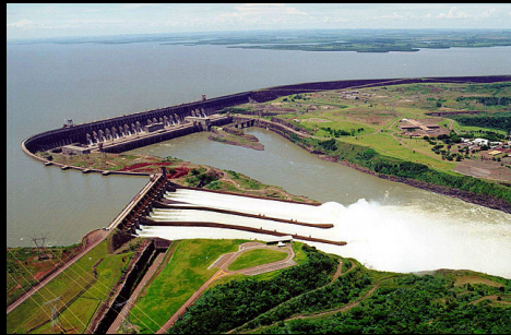
Itaipu Dam Hydro Power plant, Brazil
