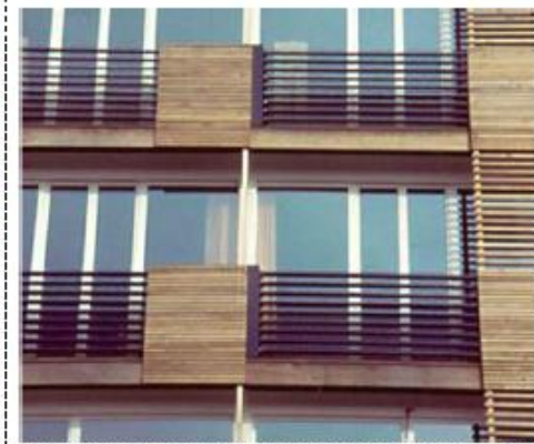
Vacuum collectors acting as balcony balustrades
